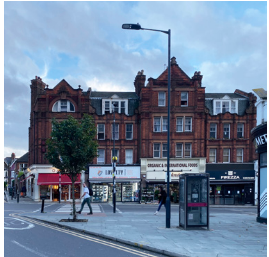
Figure 5: View from St Pauls Avenue towards Walm Lane
